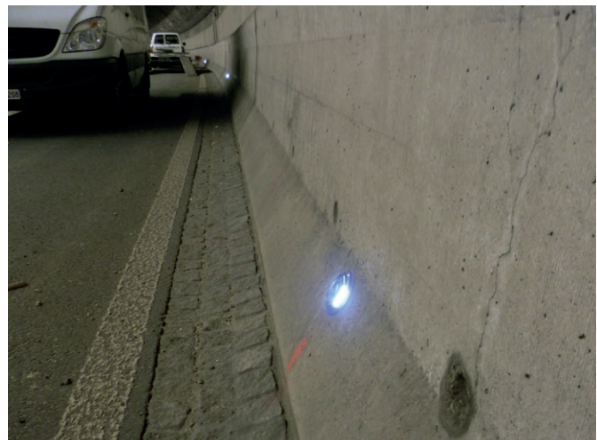
Tunnel Stephanshorn St. Gallen
